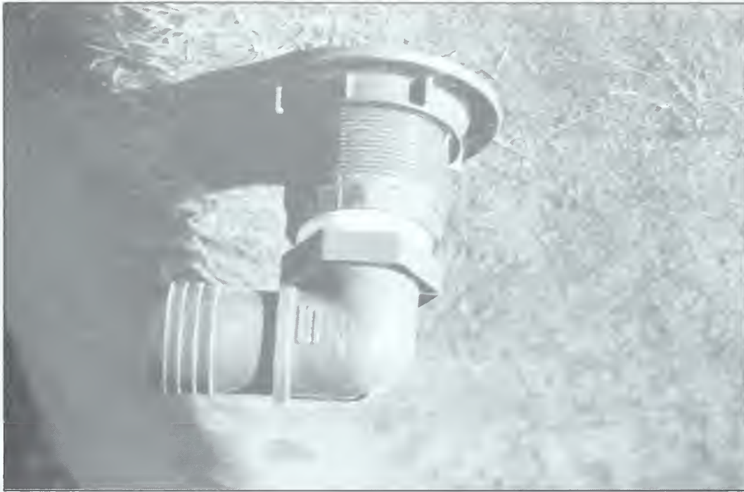
Photo 3. Bottom of fiberglass tank showing bulkhead fastener and 90° MIP-barbed fittings in place.
